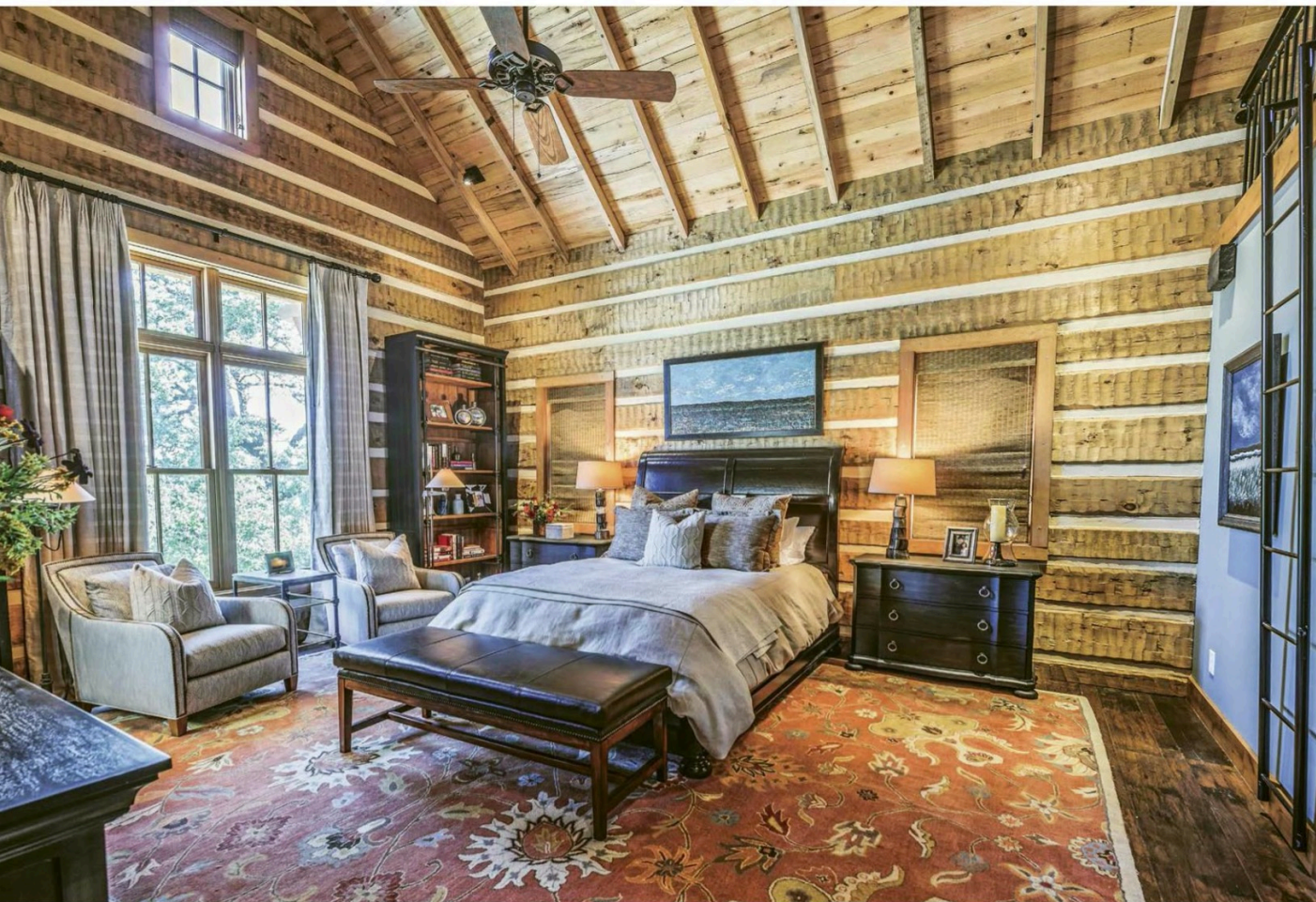
ABOVE: This 17-by-30-foot master bedroom in the main cottage has random width, kiln dried hand-hewn and distressed eastern white pine log siding on the interior and exterior. Log provider Hearthstone, Inc. mixed 8-, 10- and 12-inch widths for character and old-time authenticity. At the ridge, the room's ceiling soars 17 feet off the floor, giving the space a heavy helping of grandeur, and is encased in antique oak rafters and random-width decking in the same material. The small display loft, accessible by an iron library ladder, is positioned above the master bath.
